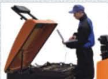
A large battery cover hood
